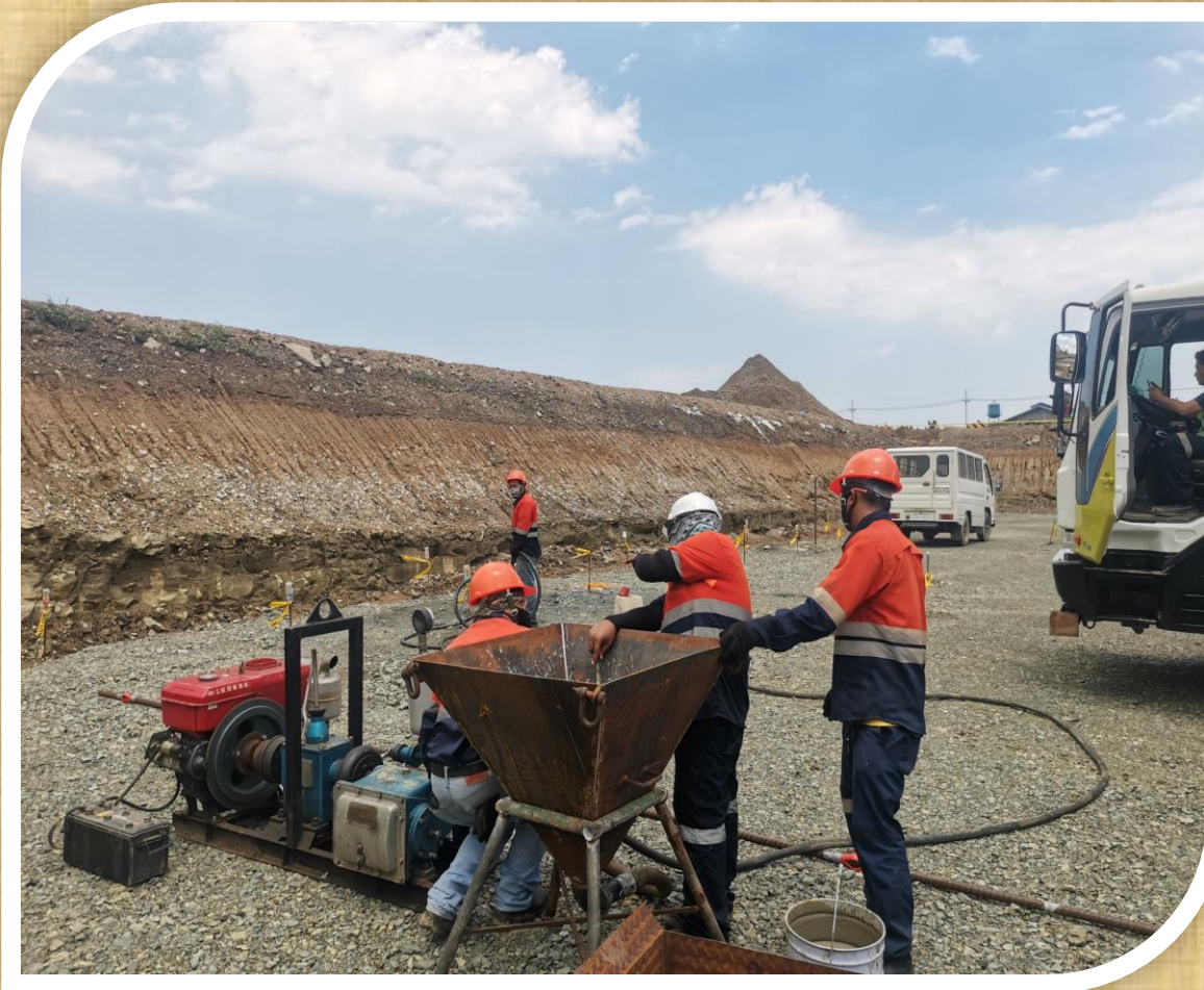
INJECTION OF CEMENTITIOUS GROUT
