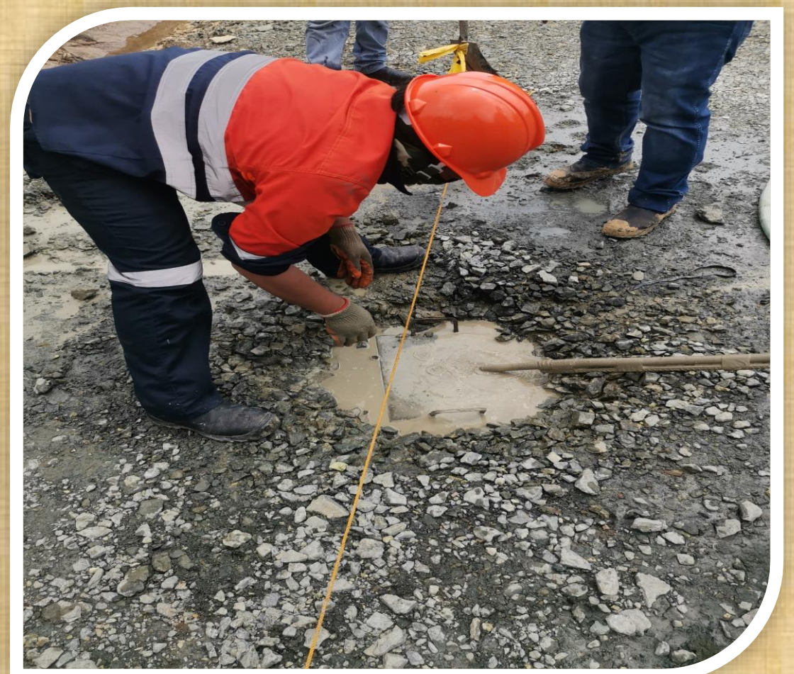
INJECTION OF CEMENTITIOUS GROUT
